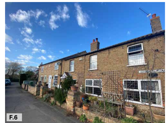
Figure 06: Historic terraced housing.
