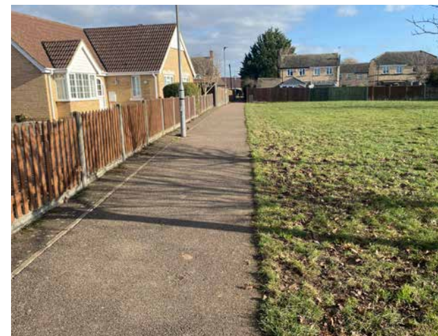
Figure 28: Footpath integrated within residential development in Wimblington offering pedestrians with onward connectivity.
