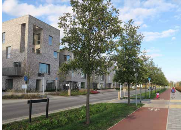
Figure 33: Example of a primary street with large street trees and green verges along the carriageway, Cambridge.
