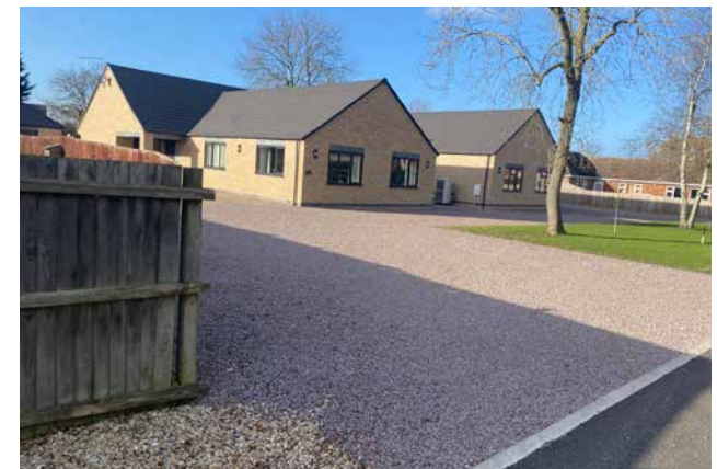
Figure 66: New large bungalow development in Wimblington.
