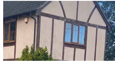
Timber framed (mock tudor)
