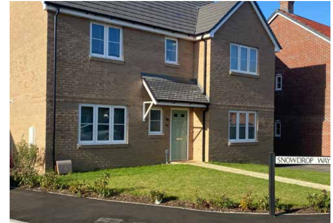
Figure 57: Grass verge and planters being used as boundary treatment.
