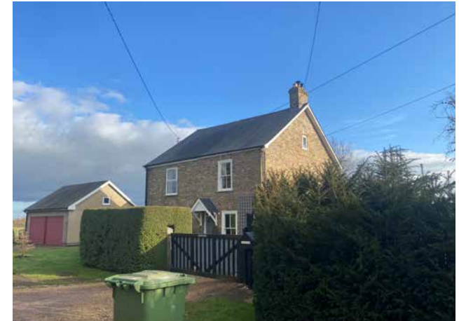
Figure 65: Traditional flat faced detached house which is found throughout the parish.
