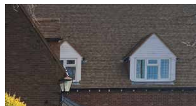
Gabled dormer with timber details
