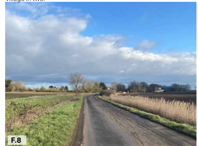
Figure 08: Rural road in Wimblington with no pavement.
