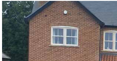
Modern casement windows
