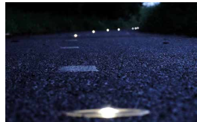
Figure 38: Example of a foot/cycle path which is lit by solar cat's-eye providing some light for pedestrian and cyclists without creating any disturbance to the nearby properties or unacceptable levels of light pollution.
